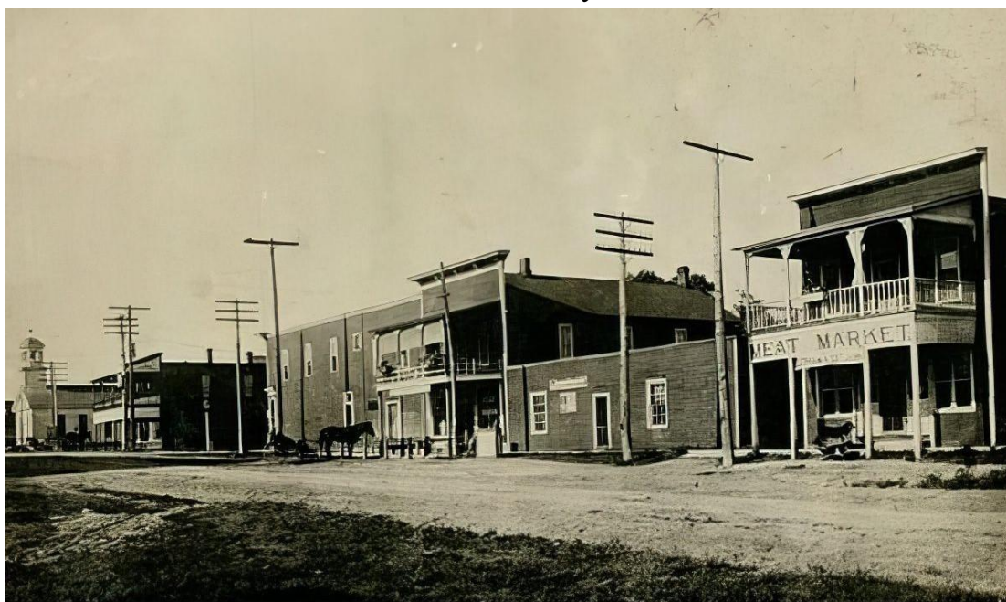
East Side of Bridge Street, 1909
