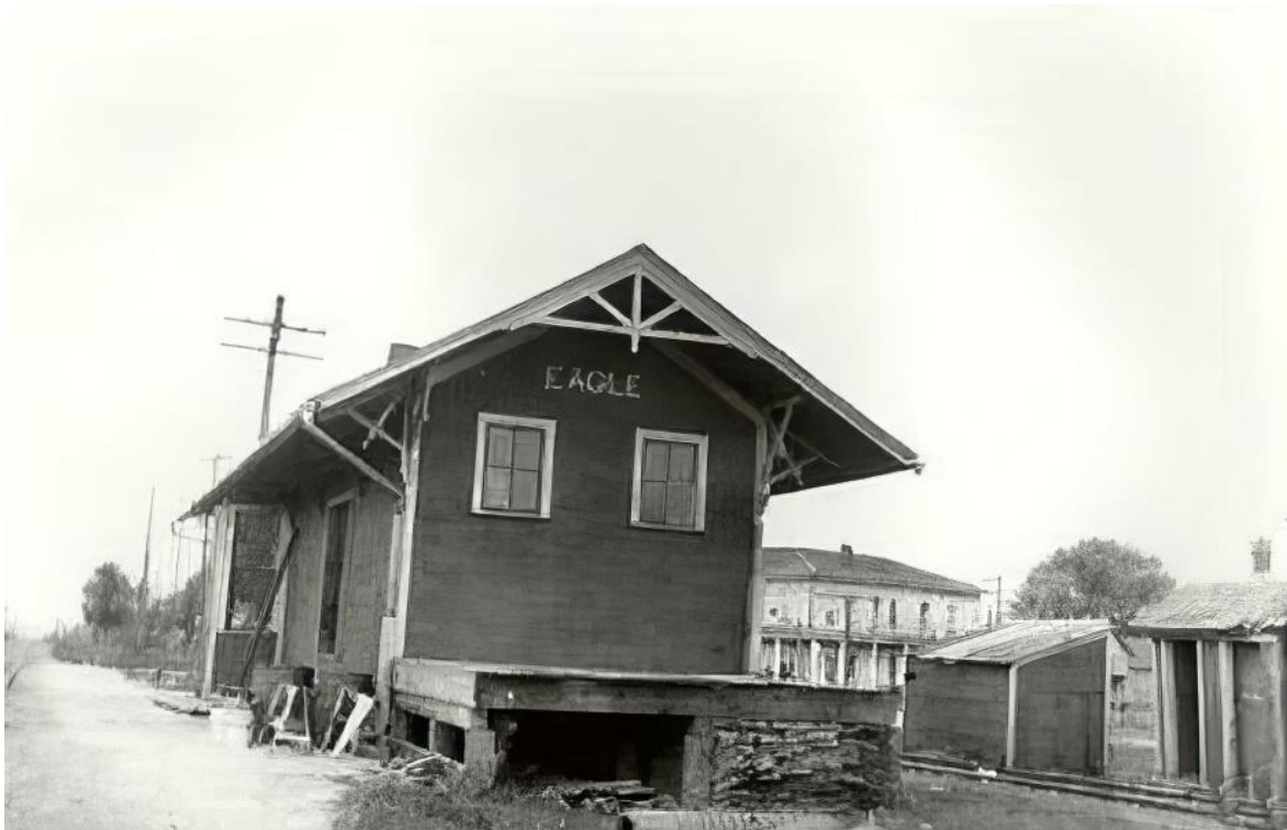
Eagle depot with hotel in background
